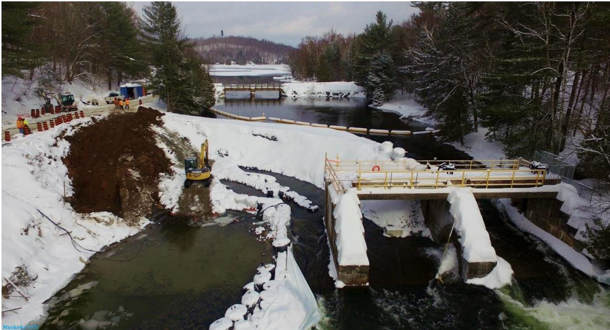
Looking upstream at Horseshoe Lake Dam construction site, February 11, 2017. Sluices 1 & 2 have been demolished.
