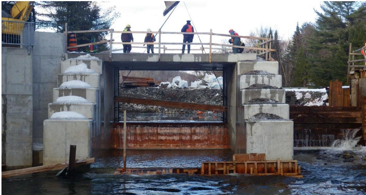
A Parks Canada engineer, dam operators, and members of the construction team are on-site as stoplogs are lowered into a brand new sluice for the first time. February 2018.
